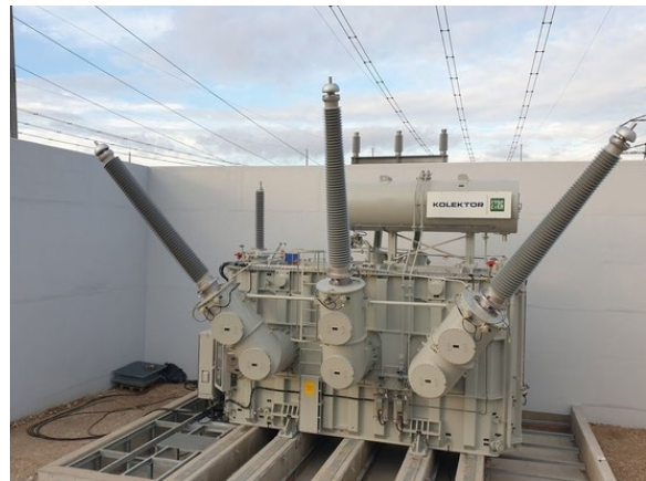
Figure 5 – 400kV Transformer
