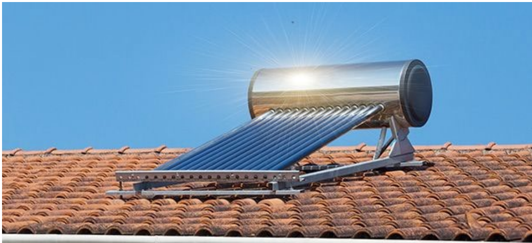
Figure 6- Solar Thermal Panels
